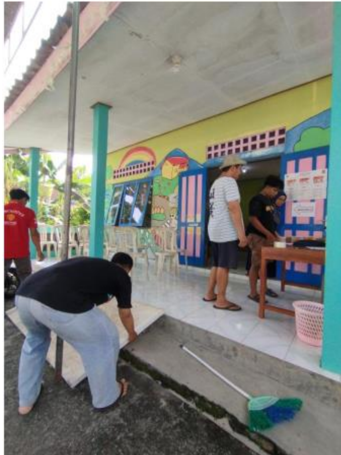
Picture 5. Installation of Boards for Wheelchair Access at TPS 02
